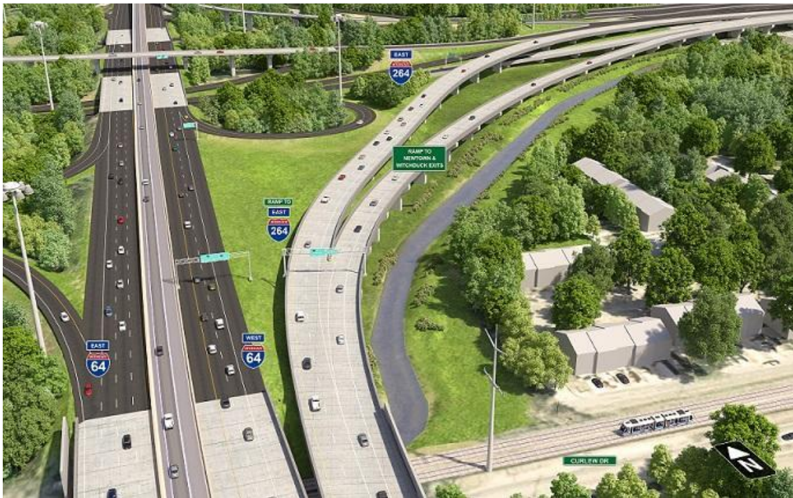
The new ramp from I-64 west to the mainline of I-264 east, shown above, opens to traffic Wednesday night.
